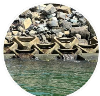
COASTALOCK Units on Harbor Island
